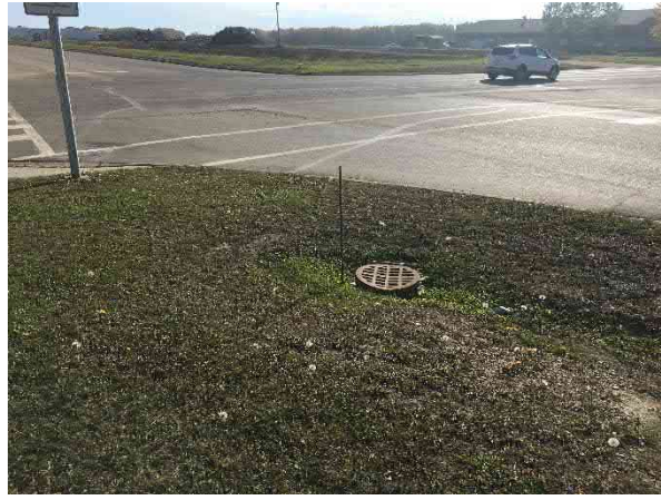
Figure 8 – Manhole in NW corner
