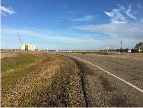
Figure 7 – Pavement sideslope at SB right turn
