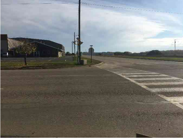
Figure 7 – Crosswalk across north leg
