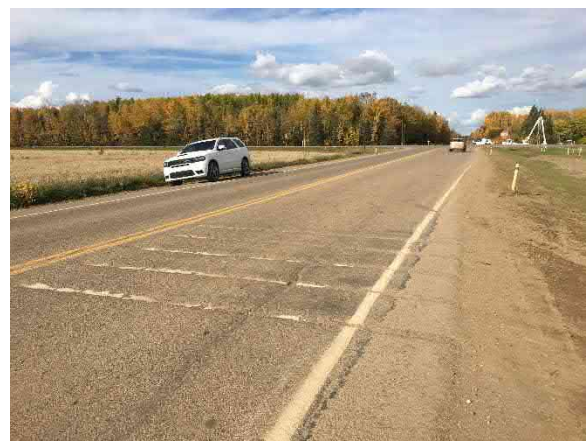
Figure 10 – Rumble strips in advance of stop
